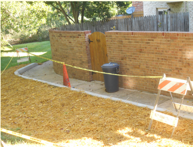
The new curb to divert excess water flow behind 7421-7429 Hallcrest Drive.
