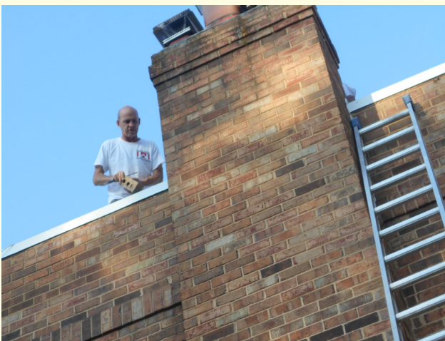
Robert Barry is our "brick expert." Here he is replacing loose bricks on the Tyler chimney.
